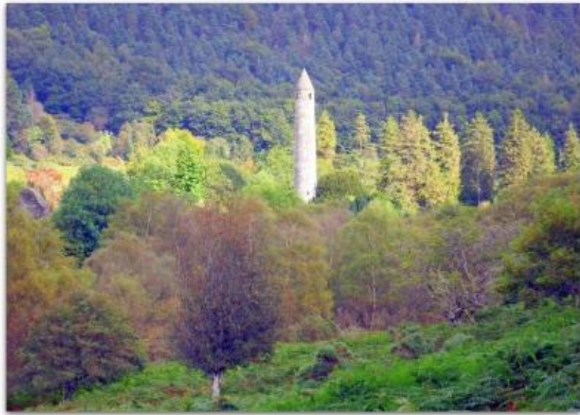
Figure 62 Glendalough, County Wicklow
