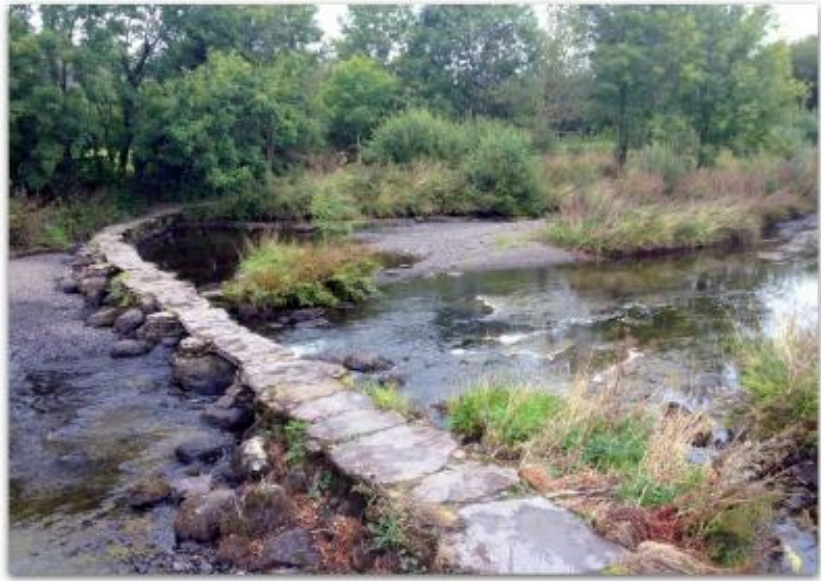
Figure 19 A Medieval "Clapper" Bridge in County Cork
