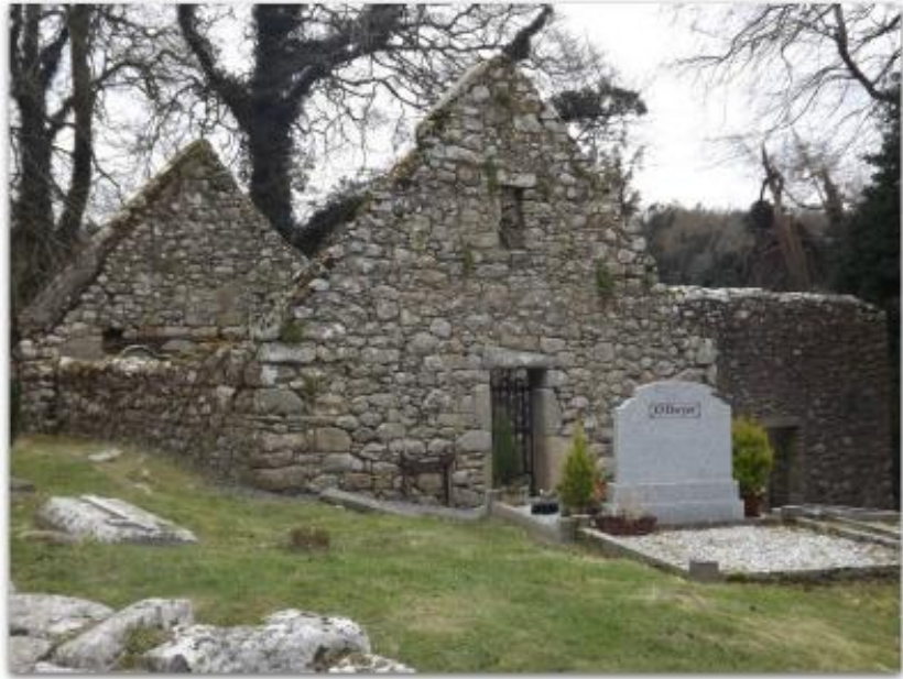
Figure 41 St. Mullins' in County Carlow
